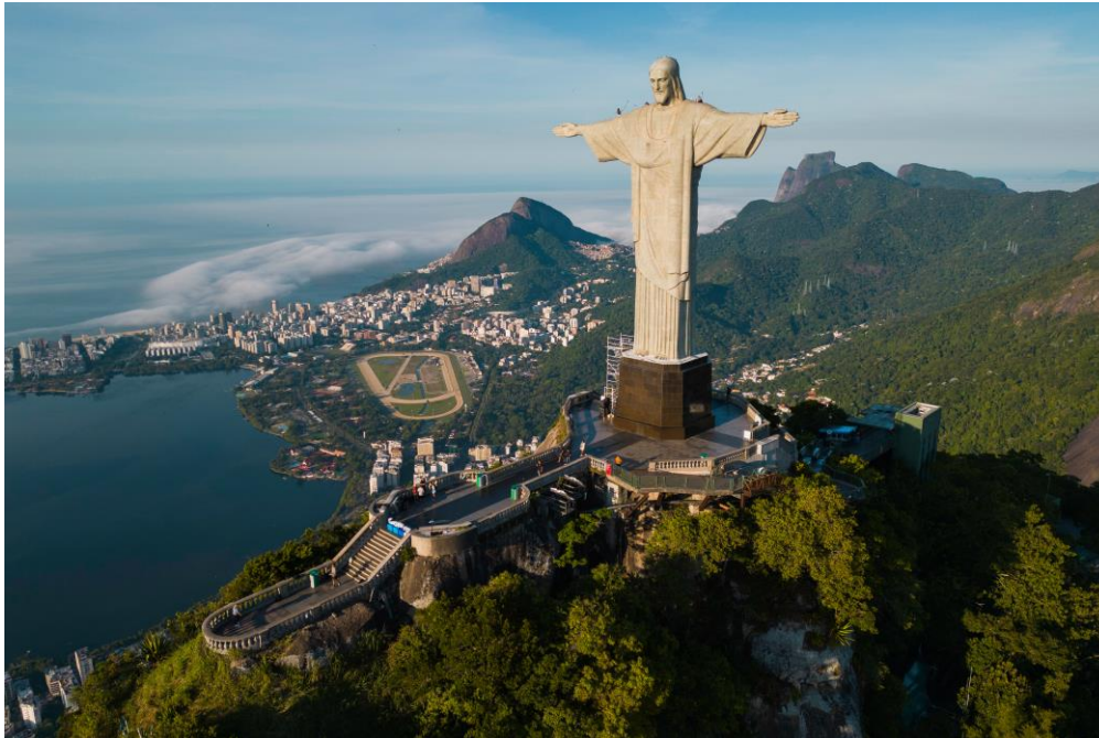
Fig 6. “Christ the Redeemer (Cristo Redentor)” 1931, Paul Landowski, Heitor da Silva Costa, Gheorghe Leonida, Albert Caquot, concrete covered in soapstone tiles, 98 feet (30 metres) tall and its arms stretch 92 feet (28 meters) wide
